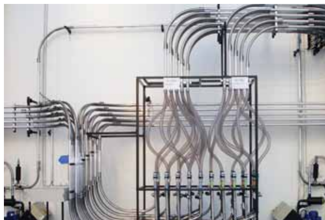
Example, Coupling station, 20 inlets/60 outlets
