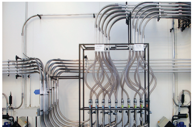
Example, Coupling station, 20 inlets/60 outlets
